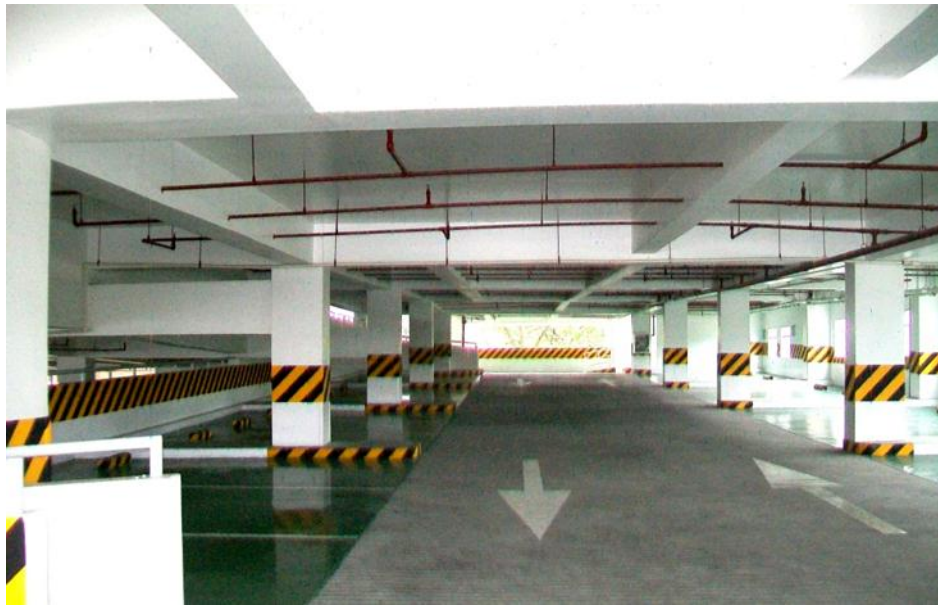
*Completed painting works
