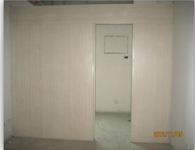
*Low partition wall installation at the 40 th floor
