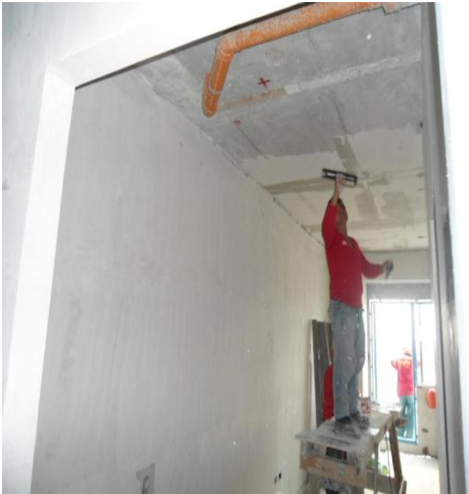
* Architectural & finishing works at 21th/27th floor
