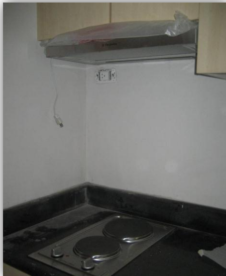
*Burner and rangehood installation at the 32 nd floor
