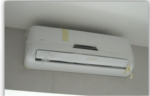
*Aircon installation at the 30 th floor
