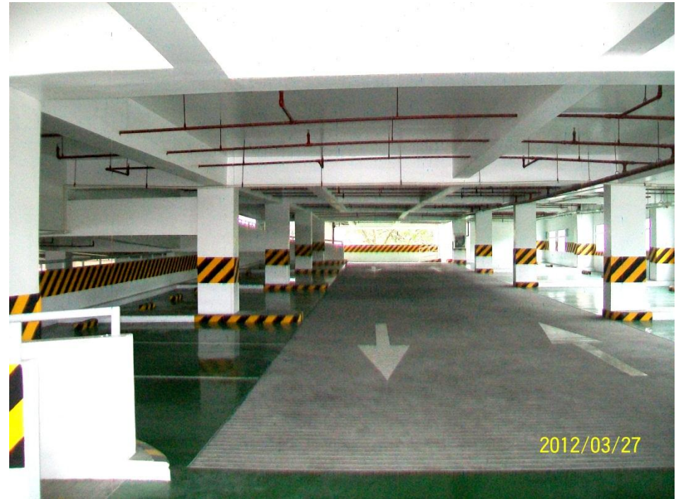
*Completed painting works
