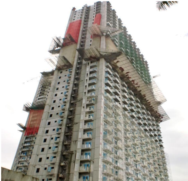
*View from Nueva Vizcaya St./ roof deck level
