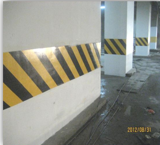
*Traffic paint at Basement 1 & 2
