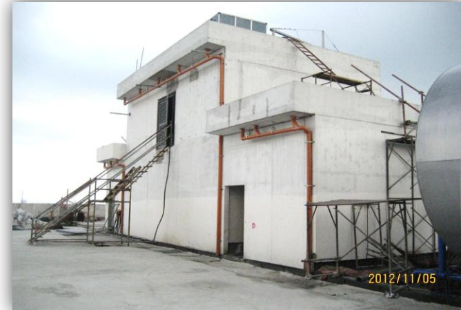
*Water tank at roof deck
